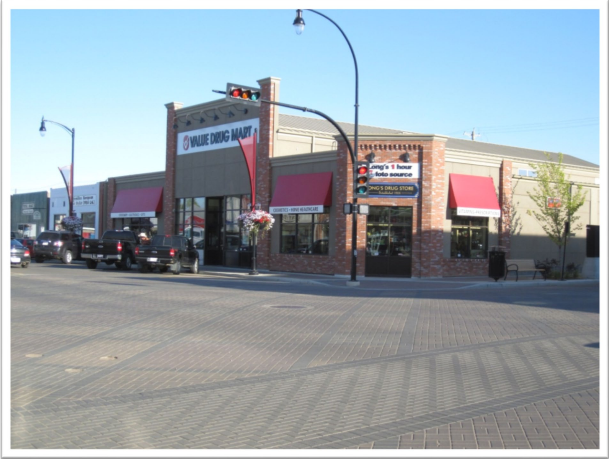
Downtown Vermilion image of streetscape improvements such as intersection treatment, tree planting and decorative light standards.
